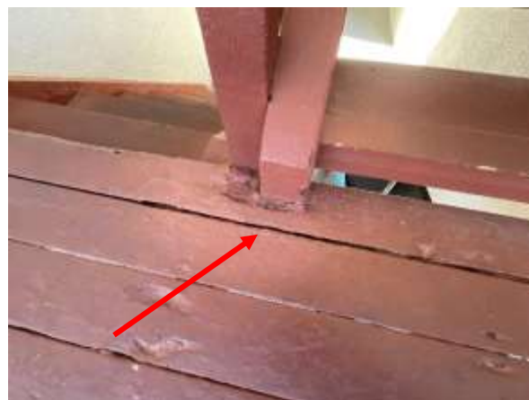
Photo 4 Stairs – Between level 1 and 2 – Overall view of unstable boards.
