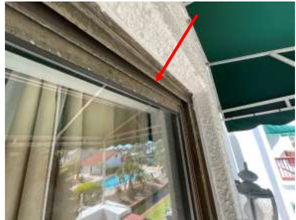
Photo 10 Private Balcony – 2 nd Floor, – Overall view of oxidation on top of sliding glass door frame.
