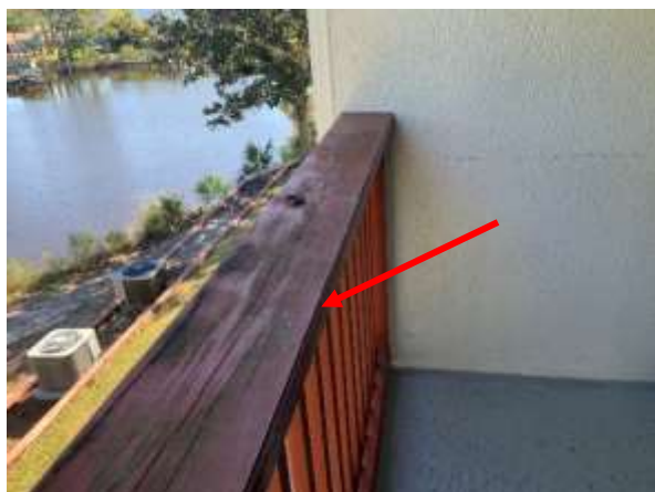
Photo 19 Private Balcony – 2 nd Floor, – Overall view of cracked and oxidated guardrail.
