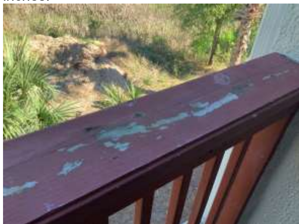
Photo 21 Private Balcony – 2 nd Floor, – Overall view of cracked and oxidated guardrail.
