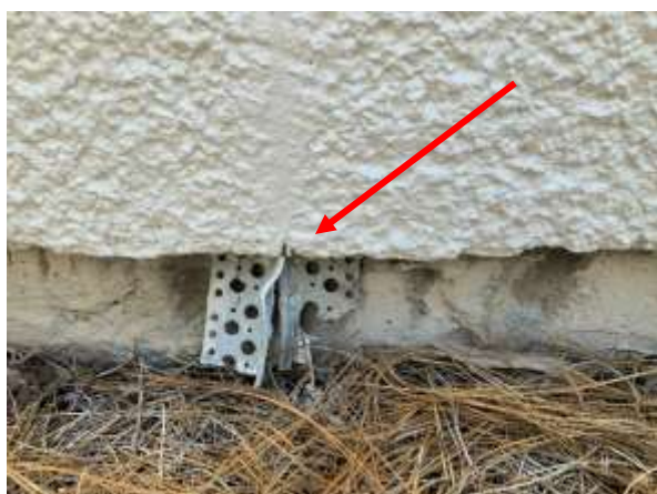
Photo 2 Base Of Wall – Ground level – Overall view of Stucco accessories at foundation.
