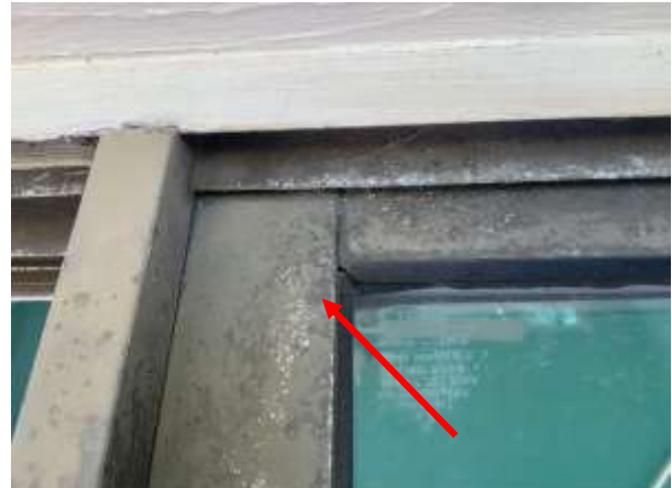
Photo 12 Private Balcony – 2 nd Floor, – Overall view of Oxidation on frame of sliding glass door.
