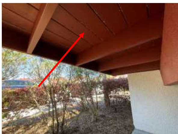
Photo 3 Stairs – Between level 1 and 2 – Overall view of unstable boards.
