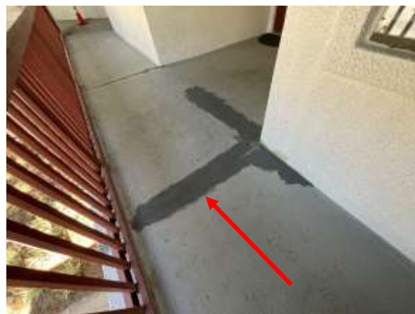
Photo 29 Common Walkway – 2 nd Floor, – Overall view of cracked and spalled concrete.
