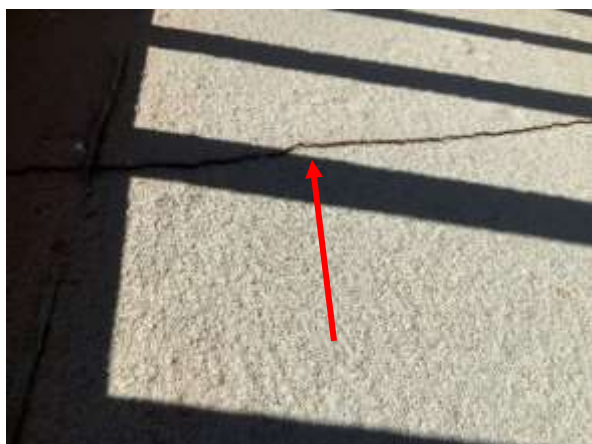
Photo 15 Private Balcony – 2 nd Floor, – Overall view of cracks and spalling on balcony.
