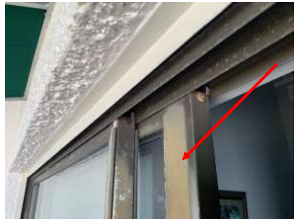
Photo 11 Private Balcony – 2 nd Floor, – Overall view of Oxidation on frame of sliding glass door.
