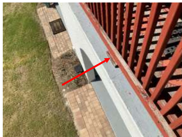
Photo 22 Private Balcony – 2 nd Floor, – Overall view of balcony guardrail sagging.
