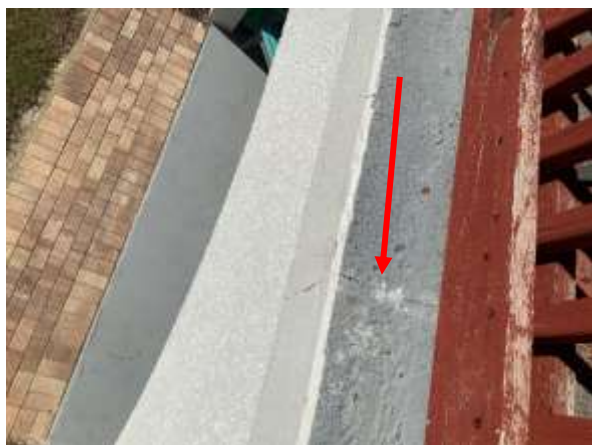
Photo 13 Private Balcony – 2 nd Floor, – Overall view of isolated cracks on balcony.
