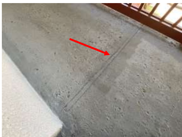
Photo 26 Common Walkway – 2 nd Floor, – Overall view of cracked and spalled concrete.
