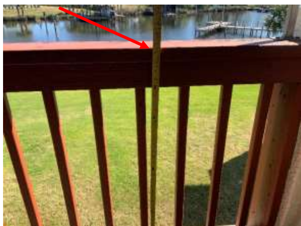
Photo 20 Private Balcony – 2 nd Floor, – Overall view of balcony height below recommended 42 inches.
