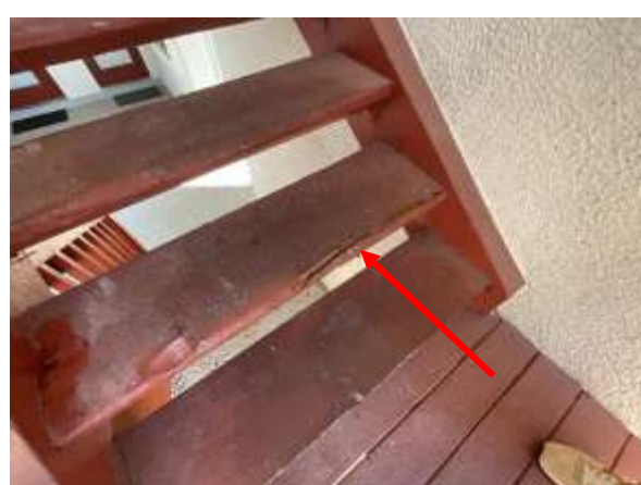
Photo 6 Stairs – Between level 1 and 2 – Overall view of unstable boards.
