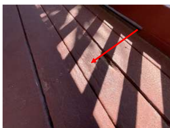
Photo 5 Stairs – Between level 1 and 2 – Overall view of unstable boards.
