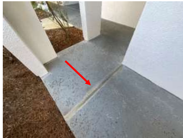
Photo 24 Common Walkway – 1 st Floor, – Overall view of failed deck coating.
