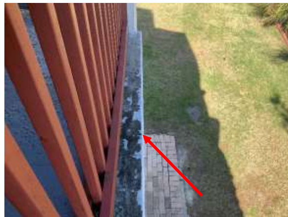
Photo 18 Private Balcony – 2 nd Floor, – Overall view of failed deck coating.
