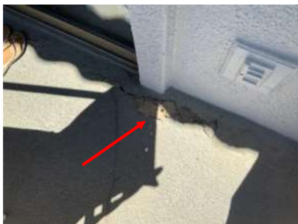
Photo 14 Private Balcony – 2 nd Floor, – Overall view of cracks and failed deck coating on balcony.
