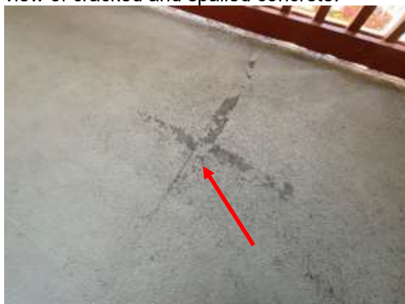
Photo 27 Common Walkway – 2 nd Floor, – Overall view of failed deck coating.
