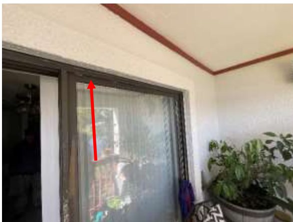
Photo 8 Private Balcony – 2 nd Floor, – Overall view of Oxidation on frame of sliding glass door.
