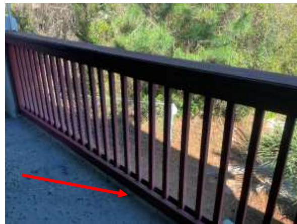
Photo 23 Private Balcony – 2 nd Floor, – Overall view of balcony guardrail sagging.
