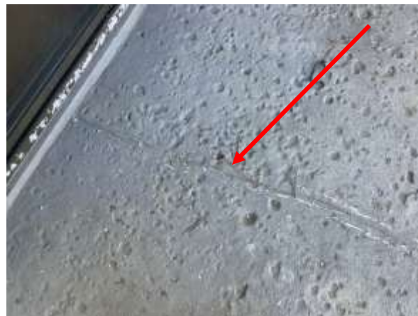
Photo 17 Private Balcony – 2 nd Floor, – Overall view of cracks on balcony.
