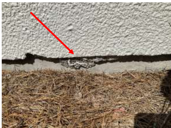
Photo 1 Base Of Wall – Ground level – Overall view of Stucco accessories at foundation.
