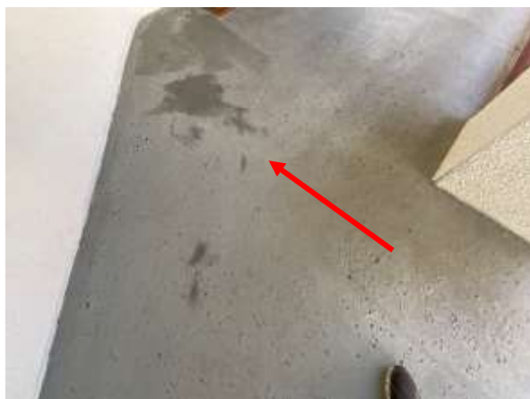
Photo 25 Common Walkway – 2 nd Floor, – Overall view of failed deck coating.
