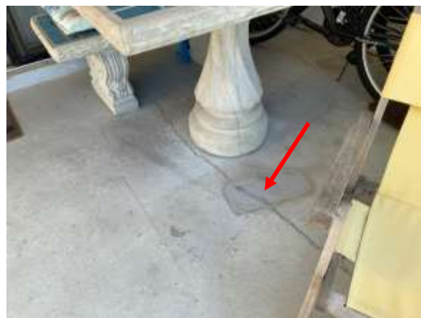
Photo 16 Private Balcony – 2 nd Floor, – Overall view of cracks on balcony.
